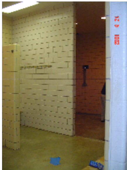
Figure 3. Shower area entry
