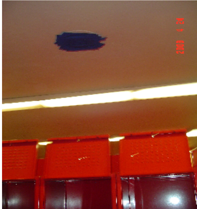
Figure 7. Setting containment. Sealing air diffusers
